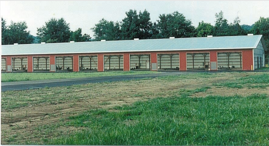
Clermont County Middle East Fork Wastewater Treatment Plant Batavia, OH — Design Flow: 7.2 MGD Waste Activated Sludge
