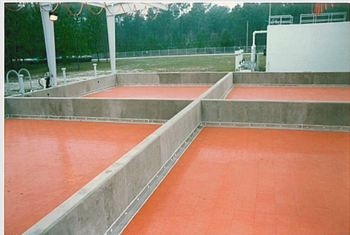
Jacksonville, Florida Naval Air Station Four 750 square foot Wedgewater™ Filter Beds Aerobically Digested Sludge
